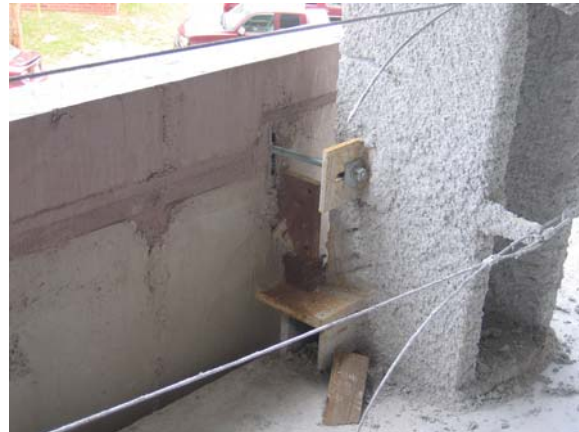
Fig 16 – Precast connections to steel columns
