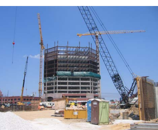
Fig 4 – Steel & Precast Erection with a view of fireproofing plastic
