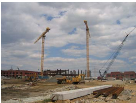
Fig 10 – Tower cranes from afar
