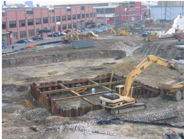
Fig 17 – Shoring for elevator pits
