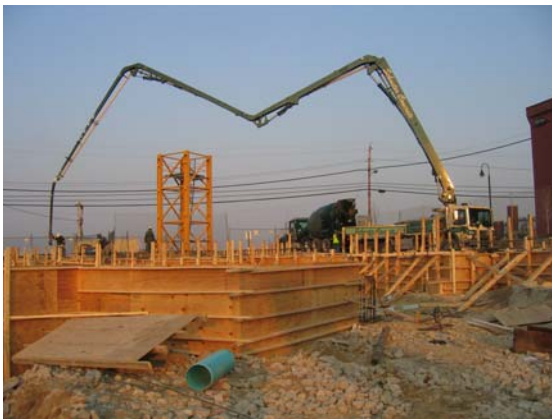
Fig 15 – Concrete Pump during foundation pours
